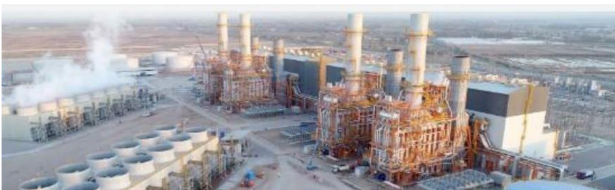
Figure 5: Photograph of a CCGT Power Plant (Nemai 2026)
